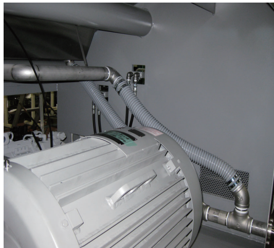
Drain inside of frame
